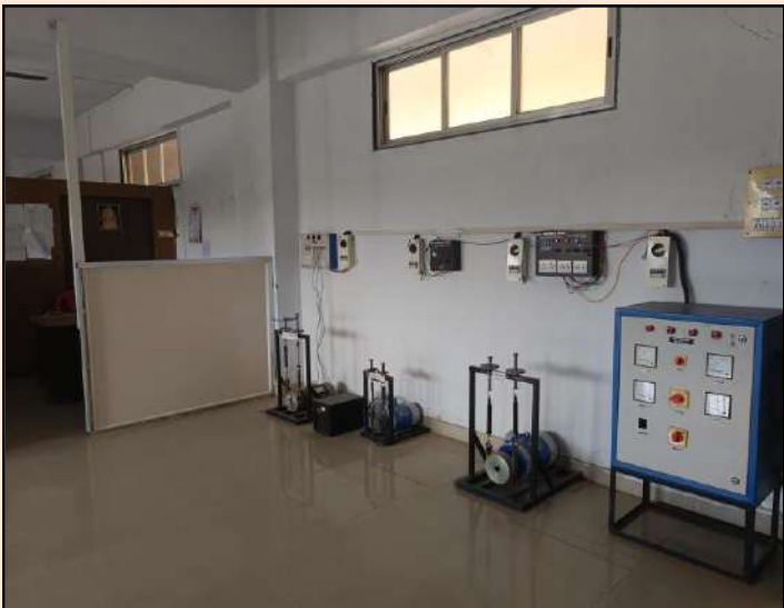
Basic Electrical Lab
